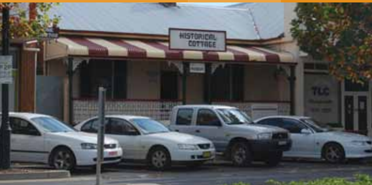
ABOVE Liverpool Plains Shire Council, Quirindi Historical Cottage and Museum Upgrade
