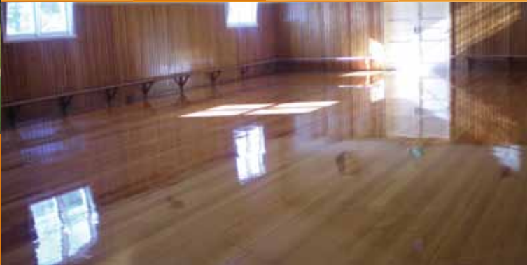
ABOVE Central Coast Council, Refurbishment of Turners Beach Hall
