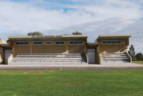
BELOW Renmark Paringa Council, Changerooms and Viewing Facilities, Renmark
