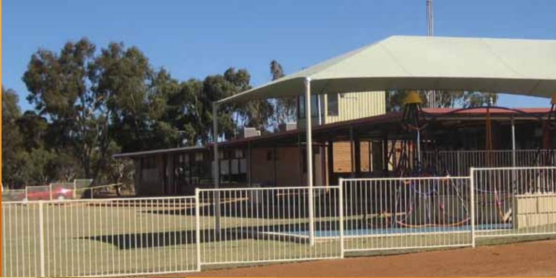
ABOVE Shire of Quairading, Playground Enhancement Project, Quairading
