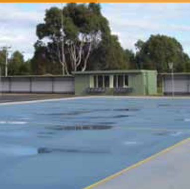
ABOVE Warrnambool City Council, Netball Courts Resurfacing
