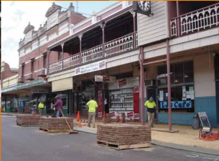
ABOVE York Shire Council, Avon Terrace Streetscape Development, York
